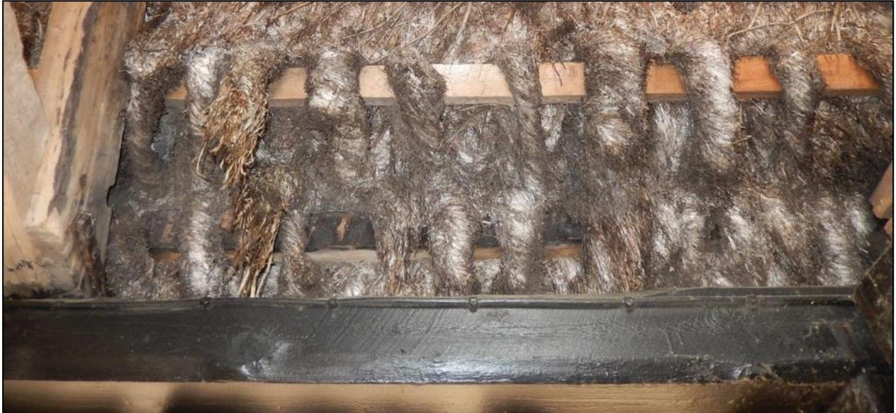
*From the underside of a seaweed roof. The 'vaskers' are bound to the lower laths.*
