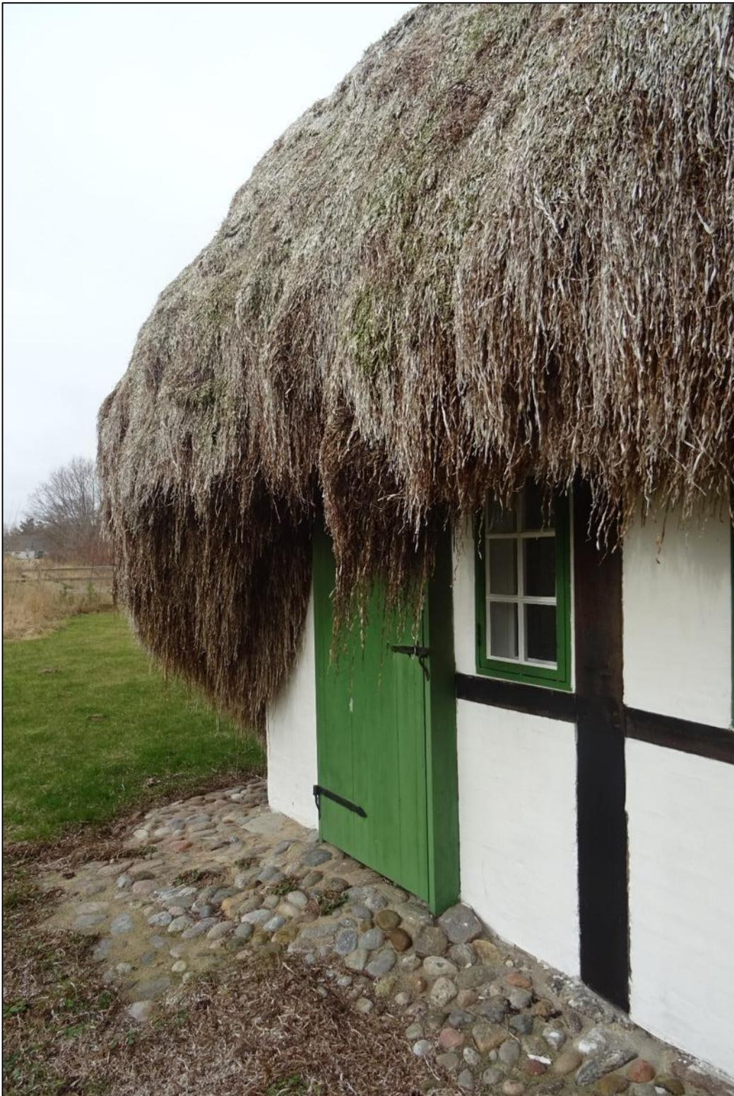
*Close-up of a seaweed roof. The stones around the house are used to lead water away from the walls.*
